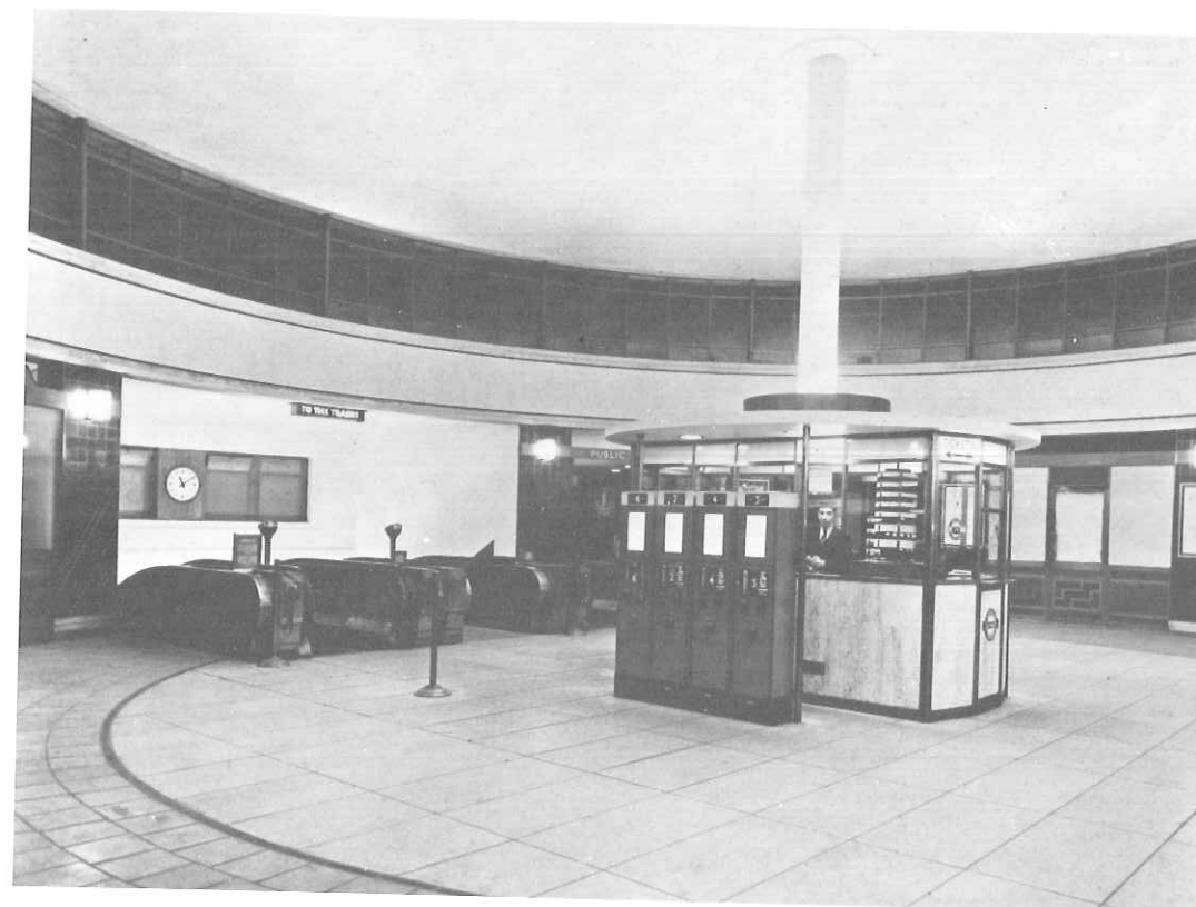
Ticket Hall, Southgate station, opened in 1933. The orderliness and unity of the design of this new station on the Piccadilly line extension contrasts sharply with the Euston entrance. The photograph is at night: in daylight the hall is lit naturally by the clerestory windows encircling the space.
